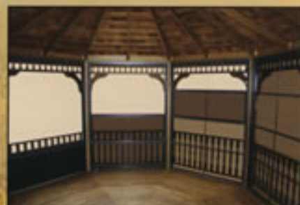
Inside View of Sliding Panels
