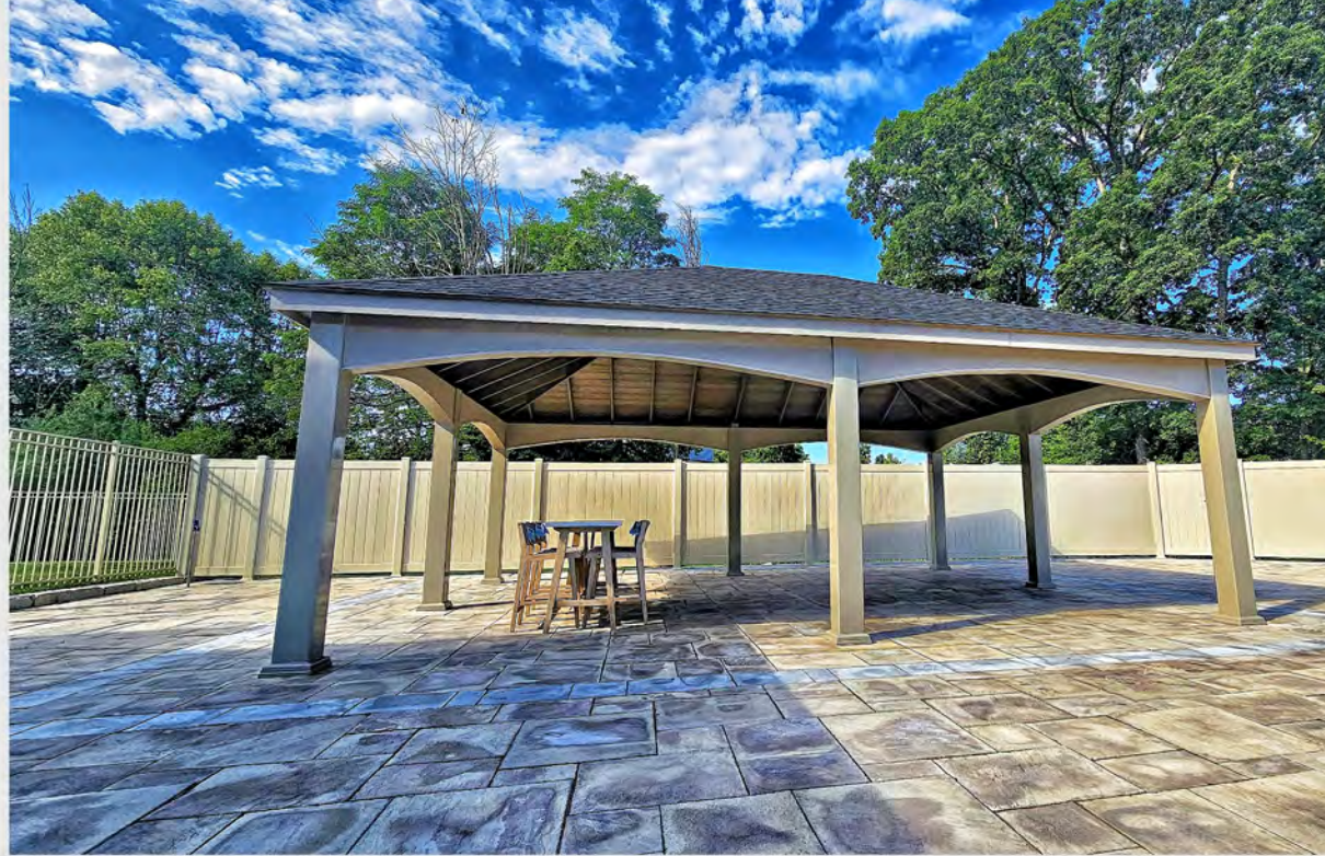
20' X 25' Clay Vinyl with Arched Headers Upgrade
