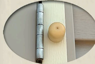
6. Stainless steel butt hinges.
