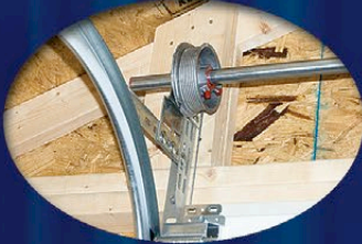
11. Torsion springs on garage doors*
