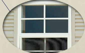
Working aluminum window, with screens and shutters.*
