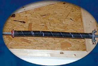
11. Torsion springs on garage doors*
