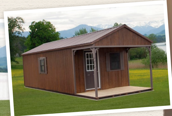
12 x 32 Custom Peak "White Deer" Cabin with porch, 9-lite house door, insulation, and other upgrades.
