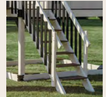
Staircase with Poly Railing
